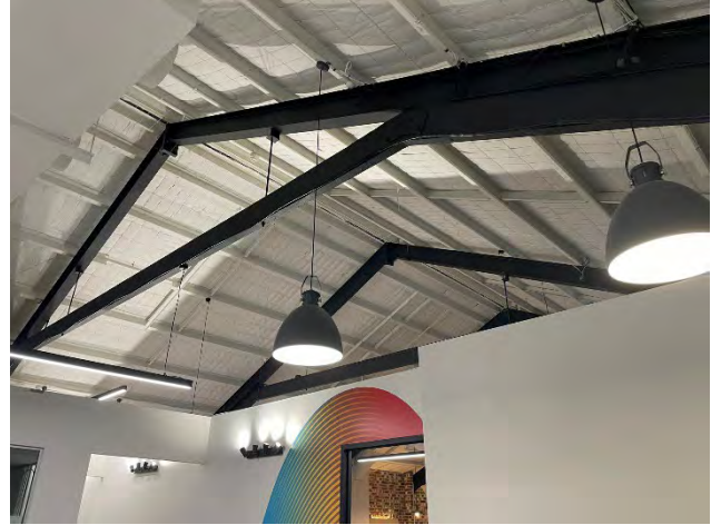
Figure 11: 19b Essex Street early timber roof truss system has been partly retained and used as a non-structural design feature.
