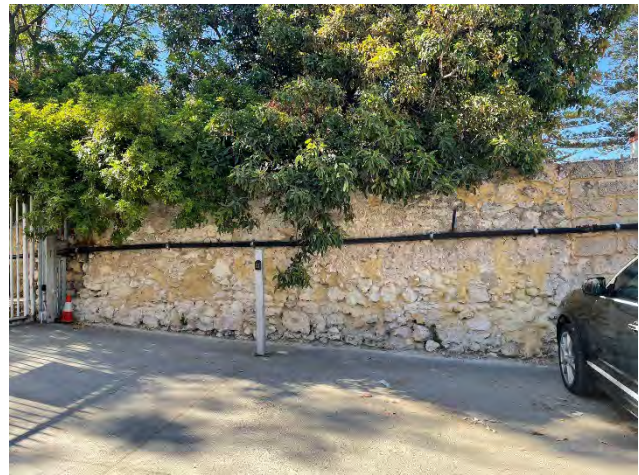
Figure 7: existing condition of the part of the boundary limestone wall to the east shared with 26-28 Norfolk Street.
