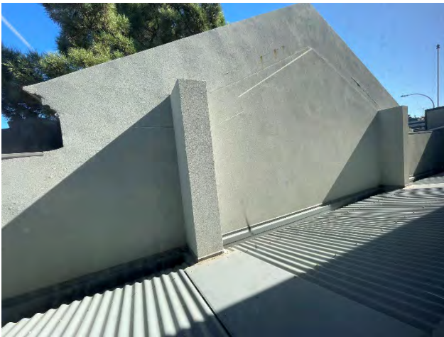
Figure 6: 19b Essex Street view behind the parapet showing skillion roof form.
