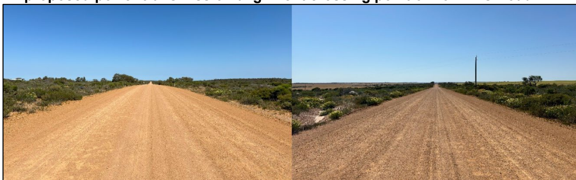
Figure 4 – View looking west and east at proposed power transmission alignment crossing point of Tomkins Road
