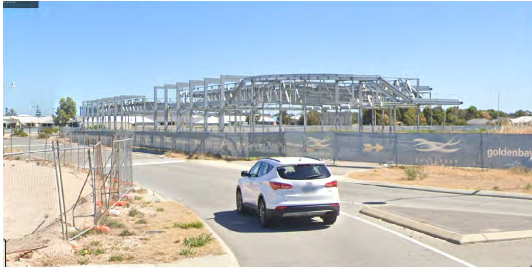
VIEW OF EXISTING STRUCTURE ALONG THUNDELARRA DRIVE
