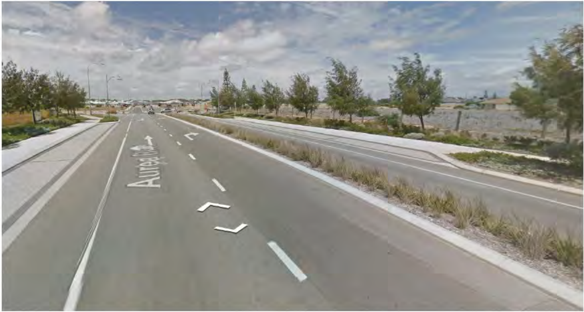
Figure 6: Aurea Blvd adjacent to the subject site (looking east)
