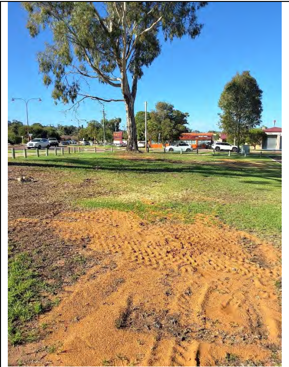
Fig. 5 - Indicating soil disturbance inside TPZ
