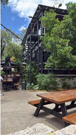
Figure 11 Parkerville Tavern south-west corner
