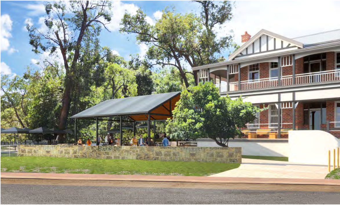
Figure 24 Oblique view from Owen Road shows alignment of horizontal elements, and the predominance of Parkerville Tavern
