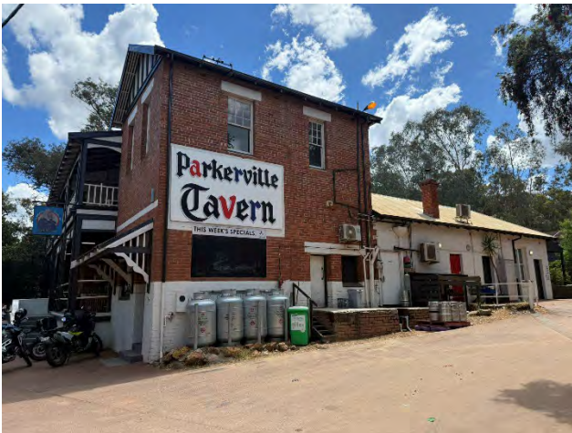
Figure 7 View from east. Left: c1926 addition Right: c1897 original Inn single storey section
