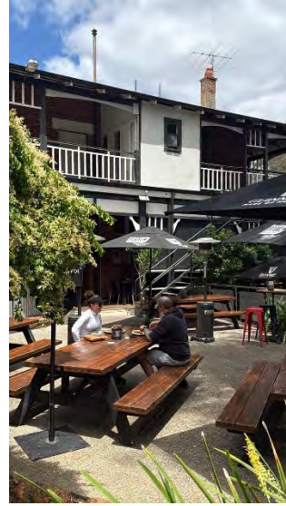
Figure 13: Parkerville Tavern West facade and courtyard
