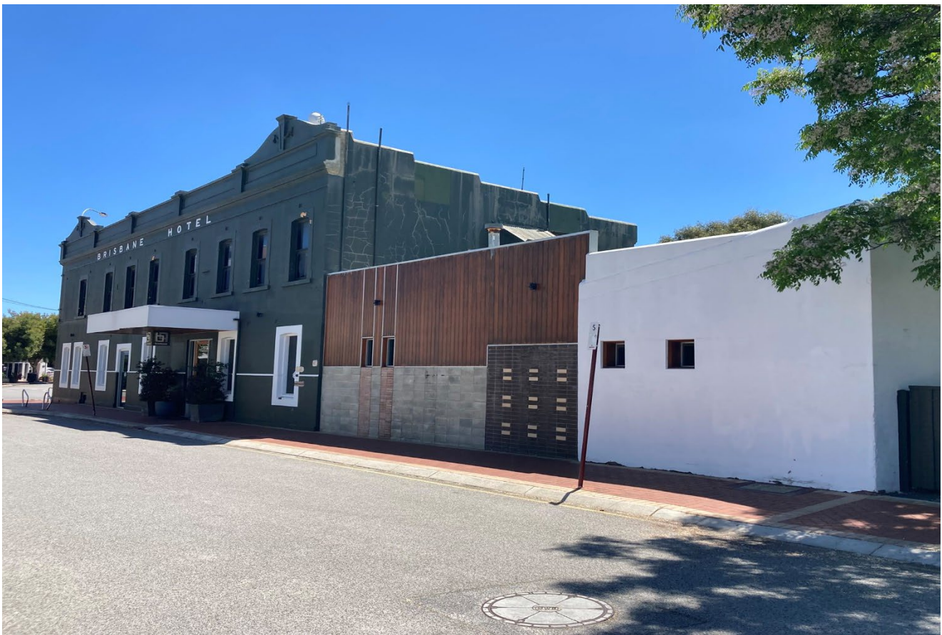
Figure 4: Brisbane Hotel, Brisbane Street looking northwards. L:1898 two storey Hotel. C: 2003 Toilet and fire escape addition, R: 2003 alterations to 1898 former Stable which now contains back of house coolrooms.
