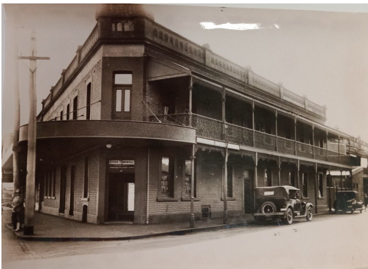
Figure 14: 1928 Historic photograph. The double storey verandah and canopy have been demolished, brick walls dado tiled and painted, and decorative facade alterations have taken place.
