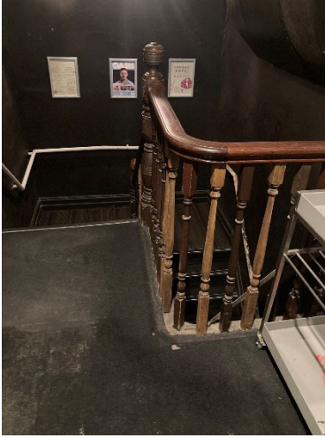
Figure 10: Staircase, with replacement timber balusters
