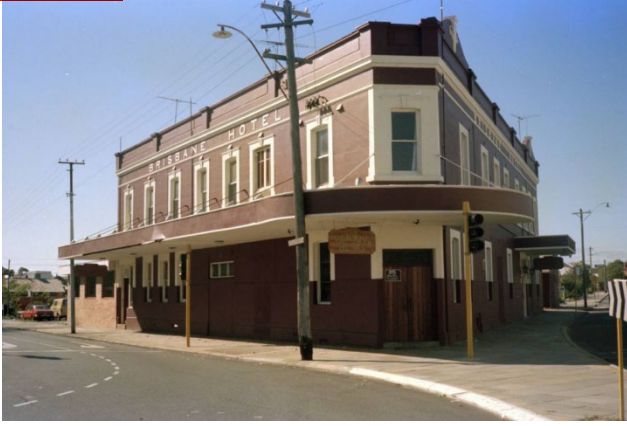
Figure 17: 1982 corner street view, Brisbane Hotel
