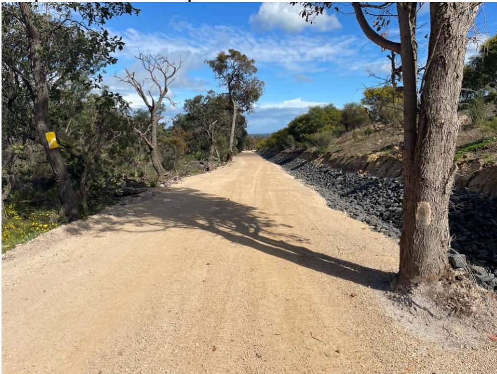
Completed Drain and Compacted Gravel Fire Track
