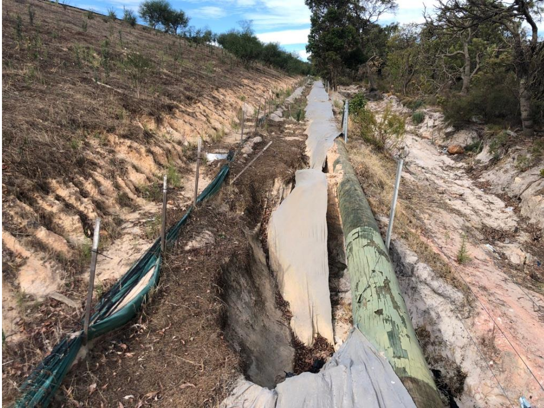
Image of failed drain flowing into adjacent fire track - Upper Section of the Drain Approximate Chainage 900 m
