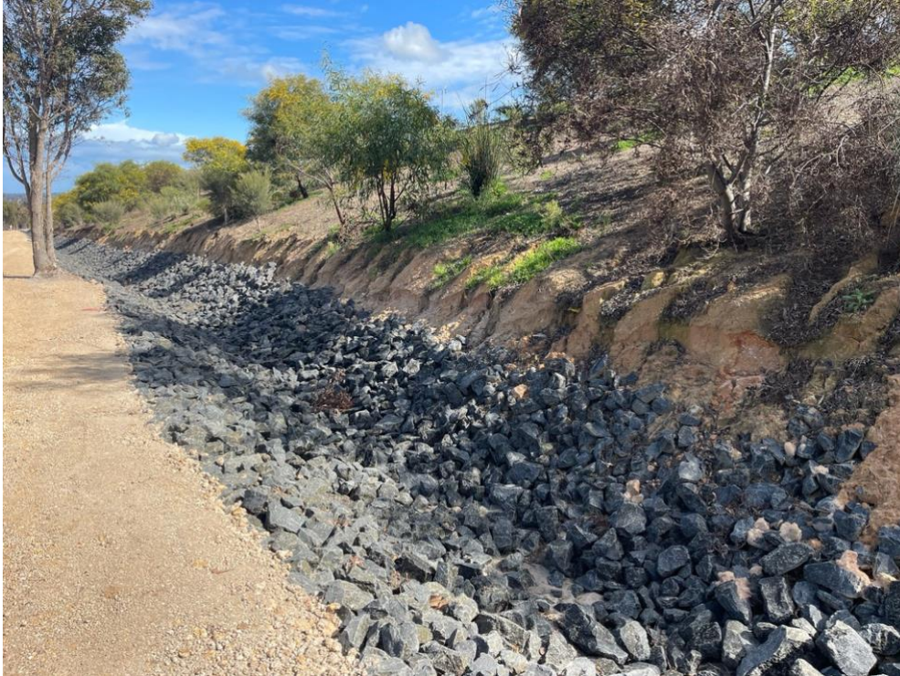
Completed Drain and Fire Track
