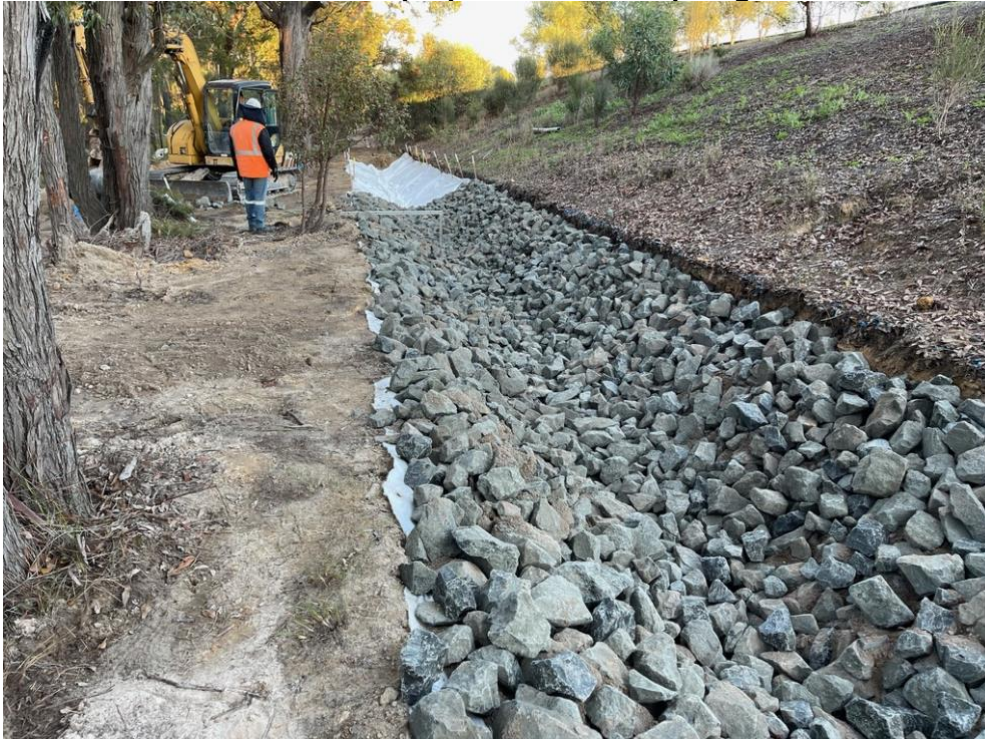
Drain Construction – Rock riprap installed on top of geotextile
