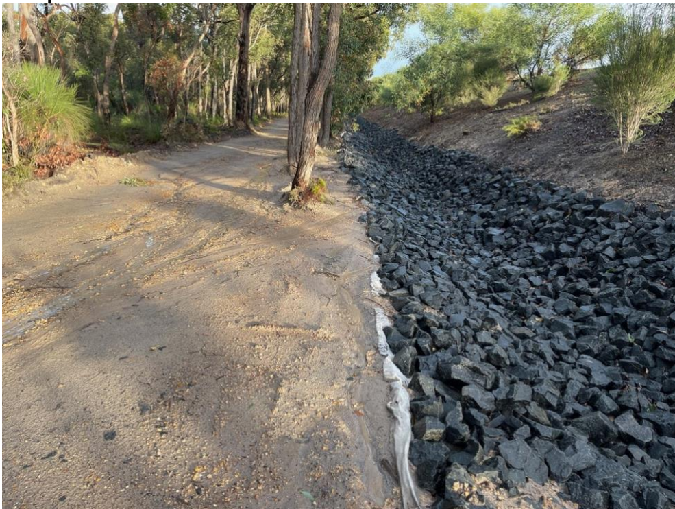
Completed Drain and Fire Track
