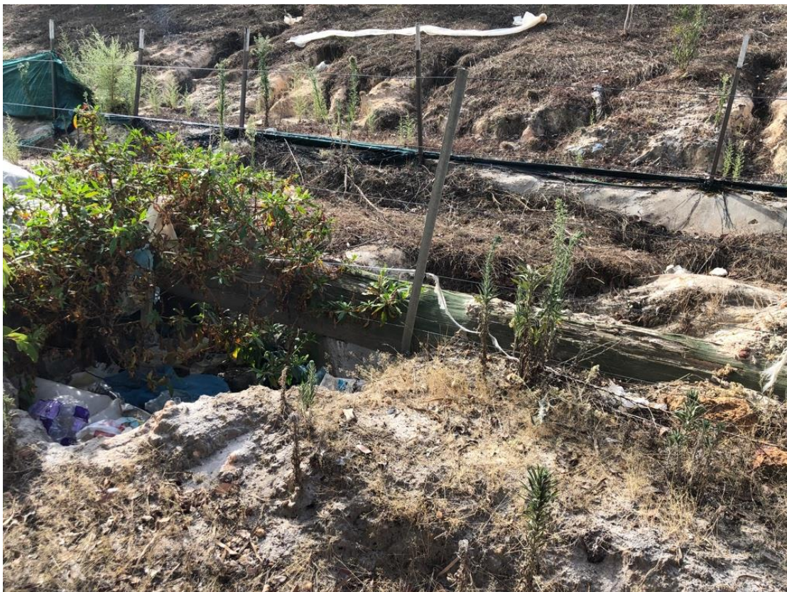
Image of failed drain flowing into adjacent fire track
