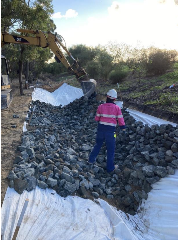
Drain Construction – Rock riprap being placed on top of geotextile
