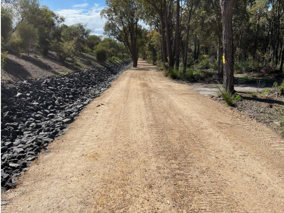
Completed Drain and Compacted Gravel Fire Track
