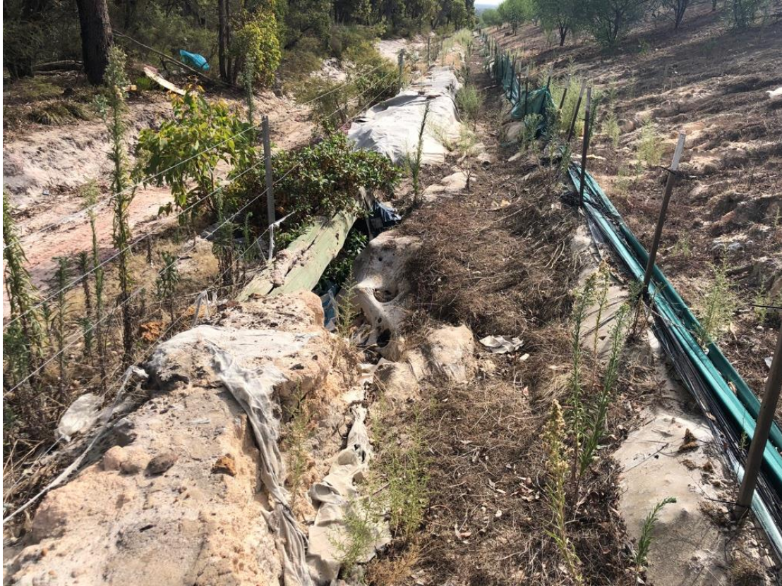
Image of failed drain flowing into adjacent fire track
