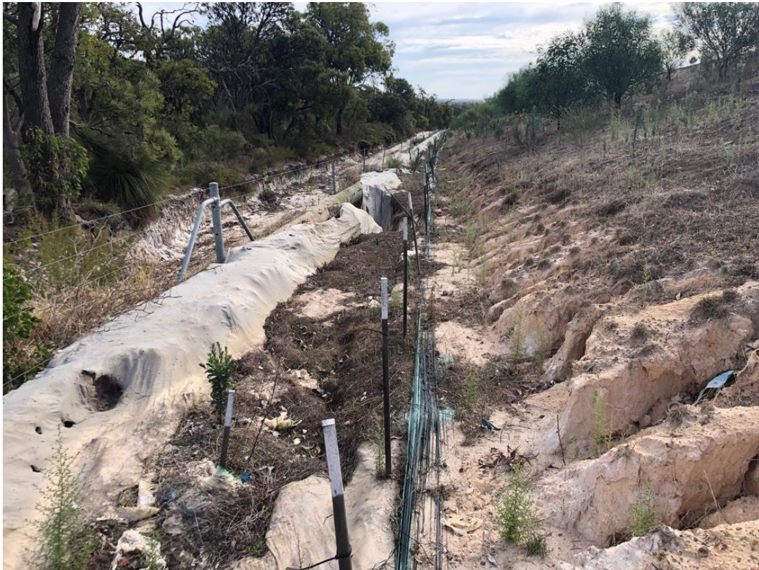
Image of failed drain flowing into adjacent fire track - Upper Section of the Drain Approximate Chainage 900 m
