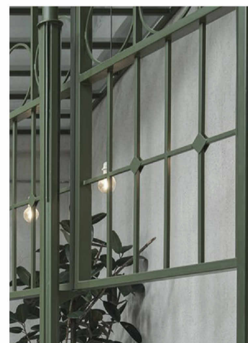
2 METALWORK FRAMING PAINTED - SAGE GREEN
