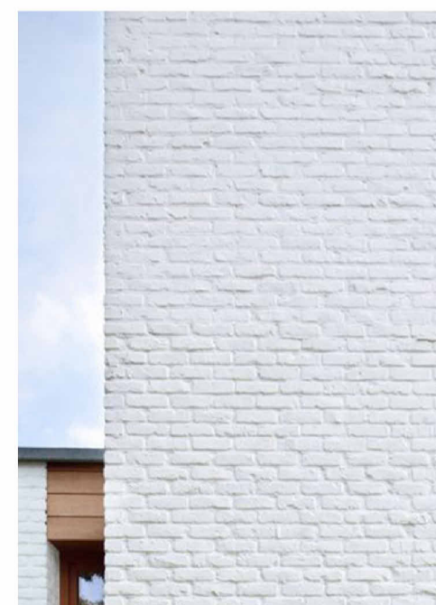
5 BAGGED BRICKWORK PAINTED - WHITE
