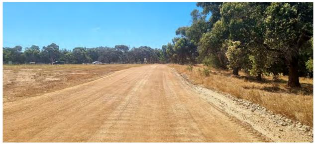
Photo 1: The operational 8 m wide construction access road adjacent to the Ki-it Monger Brook
