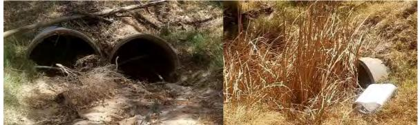
Figure 01: Existing pipe culverts, northern and southern ends respectively (extract: environmental assessment)
