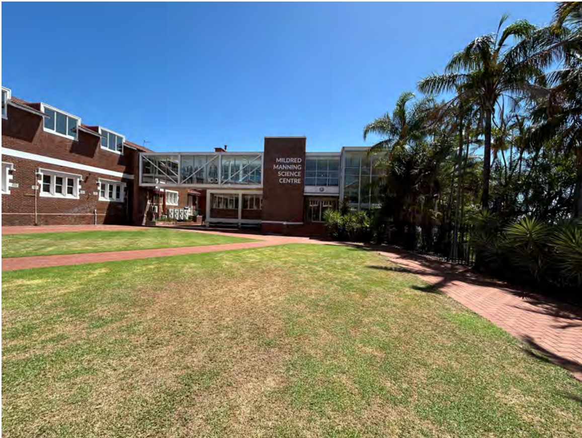
Figure 8 Looking north across the quadrangle to the Mildred Manning Science Centre.
