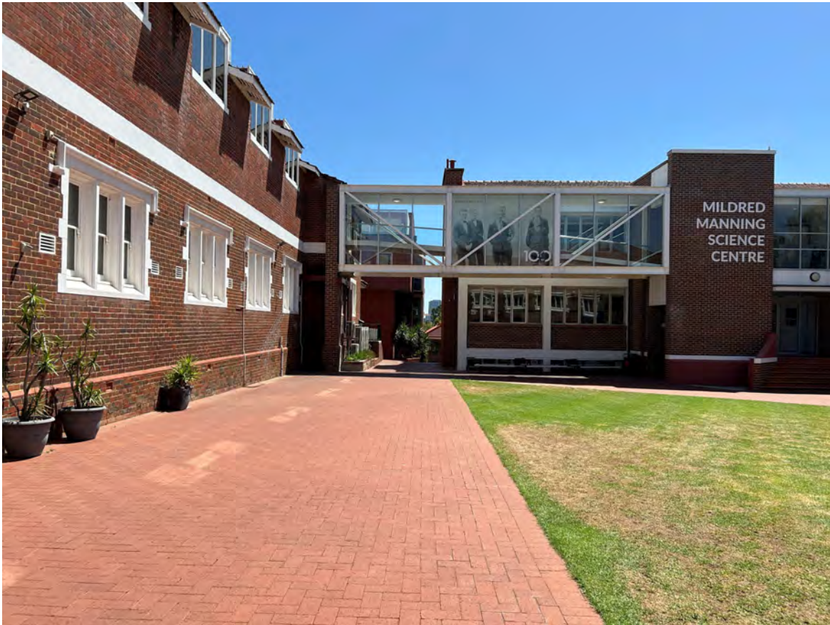
Figure 14 View across face of Trenamen Library looking north to the Mildred Manning Science Centre.
