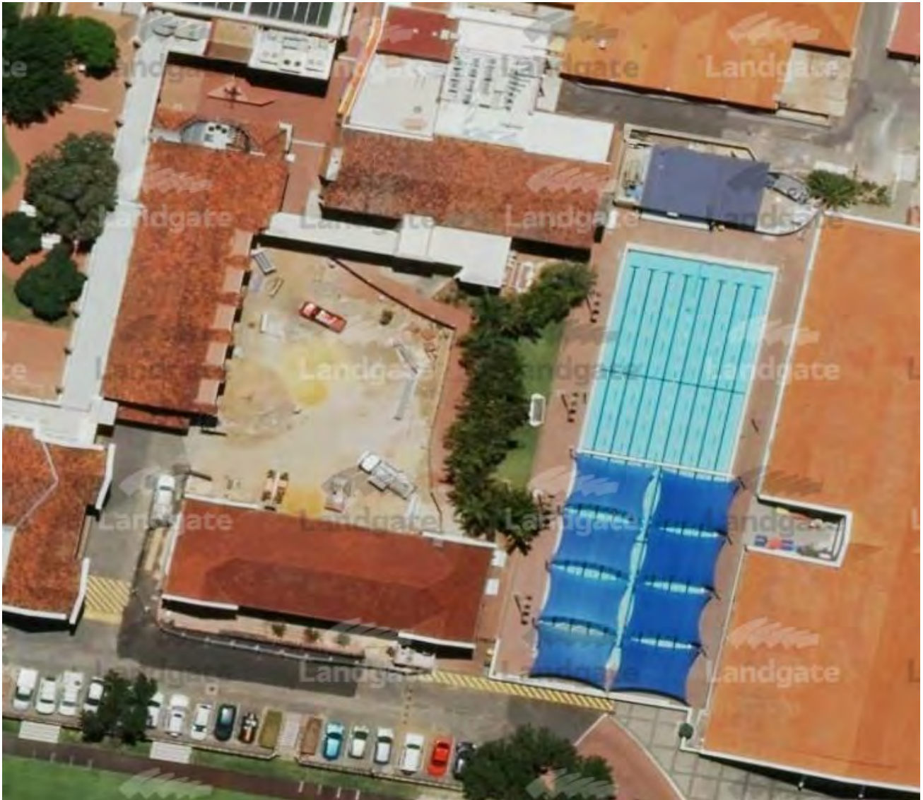
Figure 21 Aerial photographs of the site, January 2018 showing the ground works over the site. Courtesy Landgate
