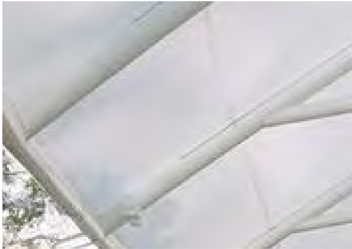
Painted Steel Members
