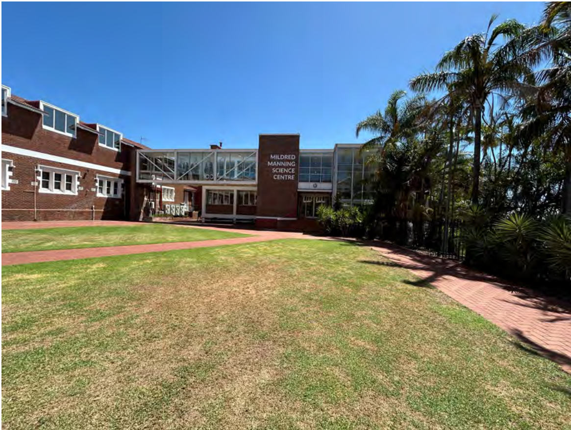
Figure 16 View across quadrangle to Mildred Manning Science Centre.
