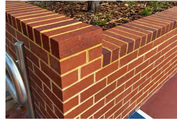
1 RED BRICK WALL
