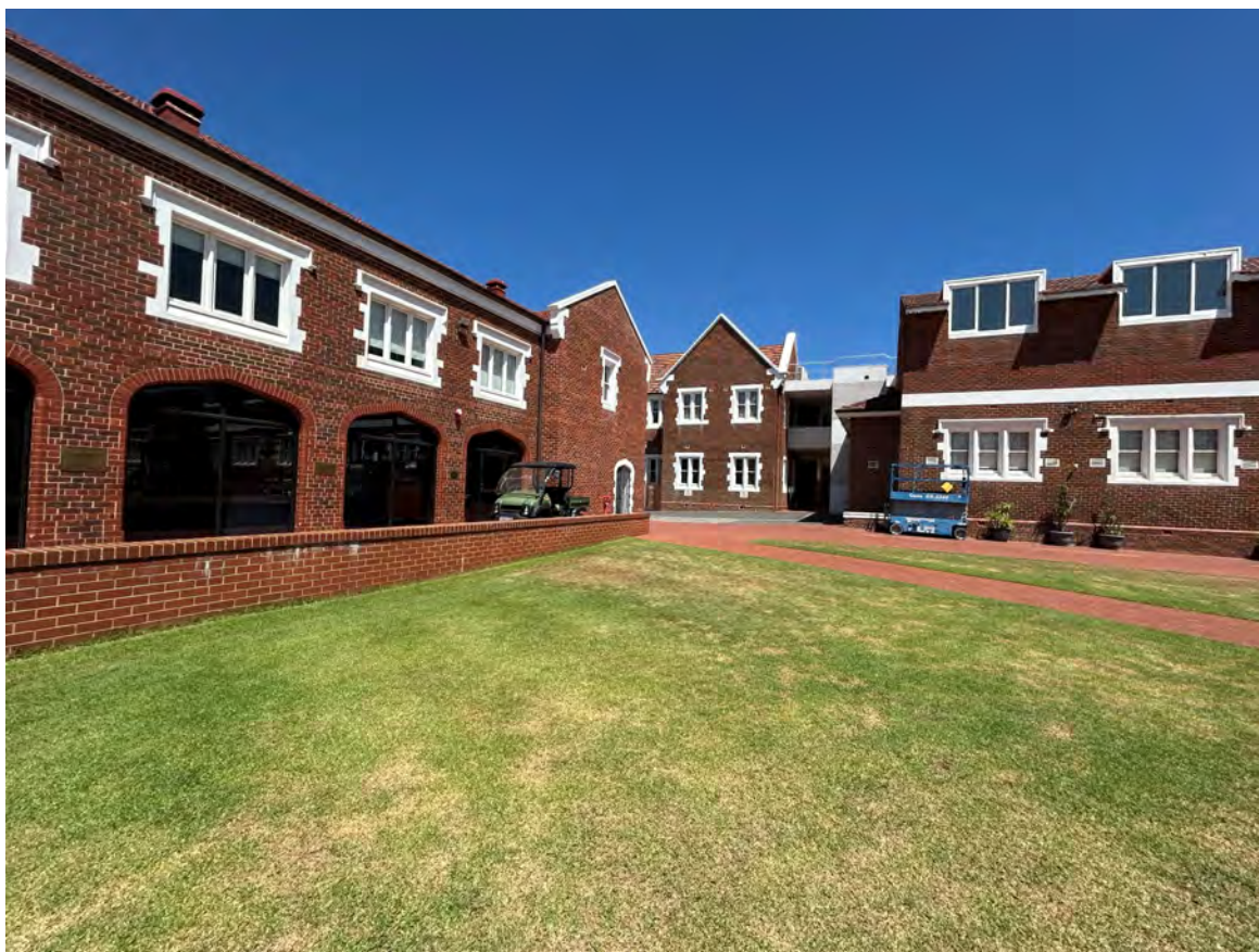
Figure 12 Southwest corner of quadrangle showing Kefford Wing identified of Heritage value beyond.
