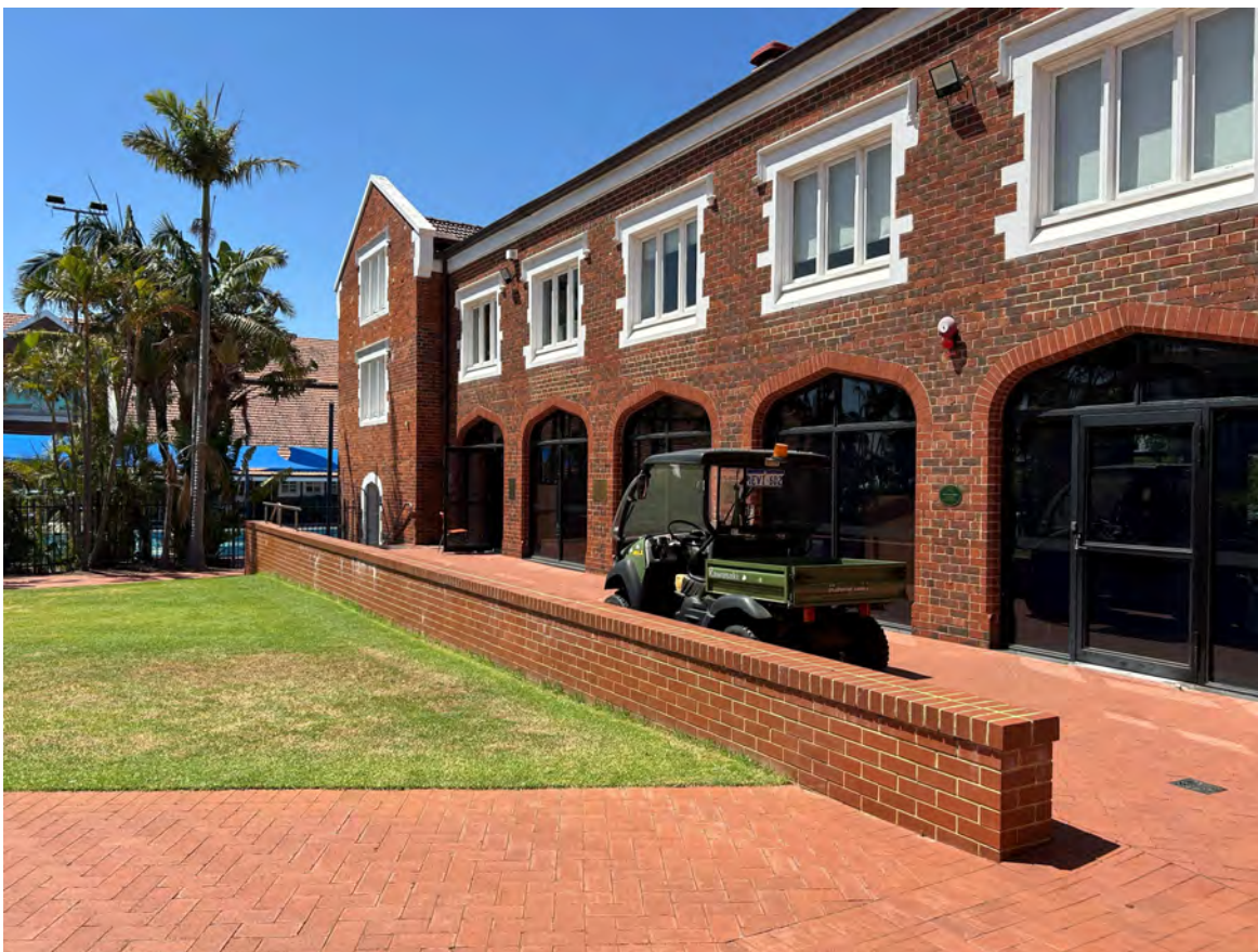
Figure 9 Hamer Wing and retaining wall to be removed.
