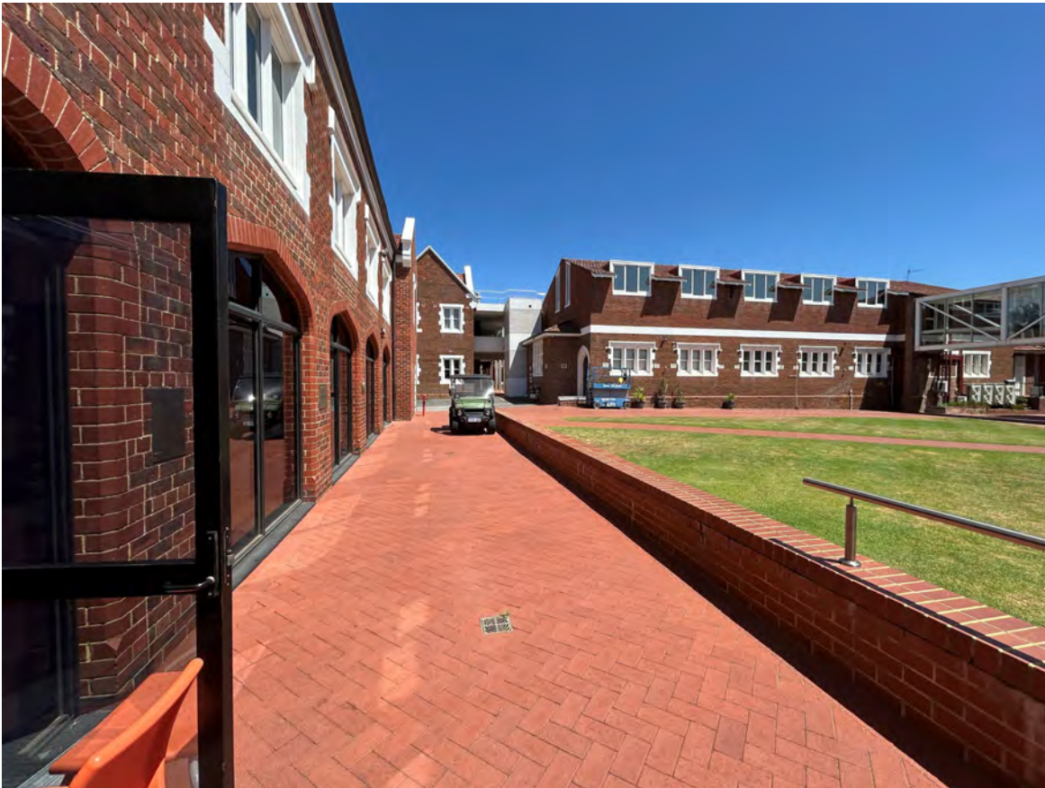
Figure 10 View across face of Hamer Wing to west.
