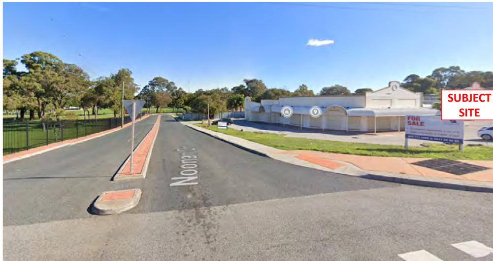
Figure 4. Westbound view along Noonan Drive from Wanneroo Road
