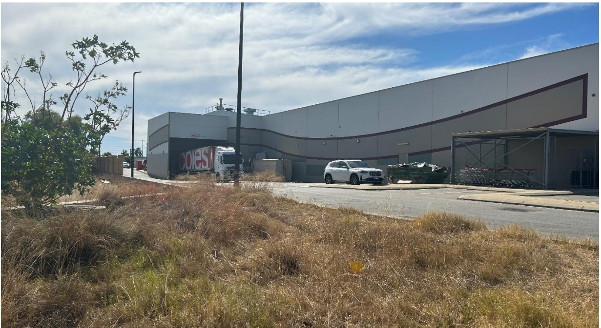
Figure 4 - Coles Supermarket Loading Dock
