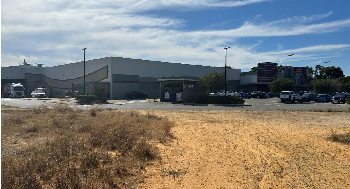
Figure 5 - Existing Bin Storage Structure
