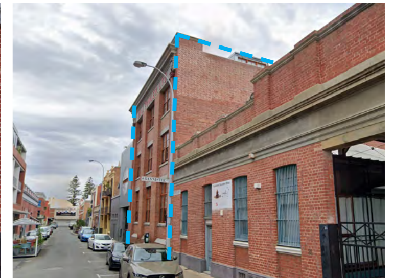
Looking at 33 Pakenham St.
