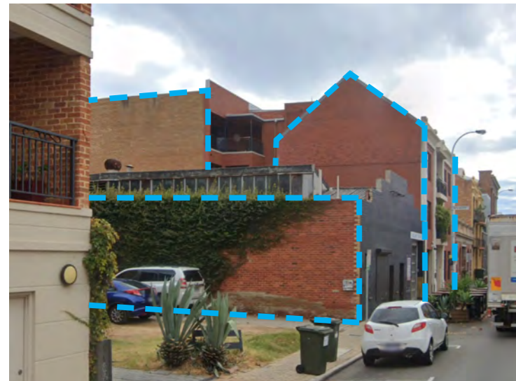
Looking at 47 & 45 Pakenham St.
