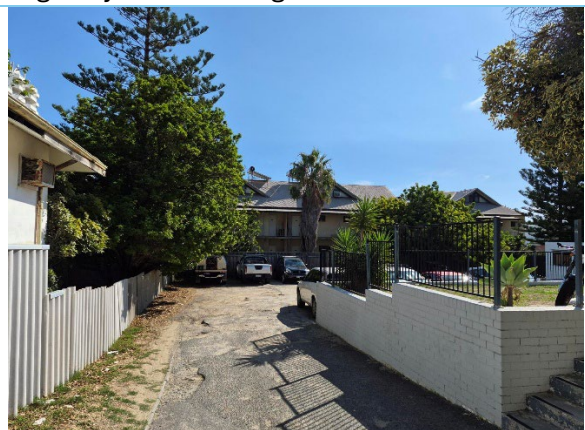
View of property from east (rear)
