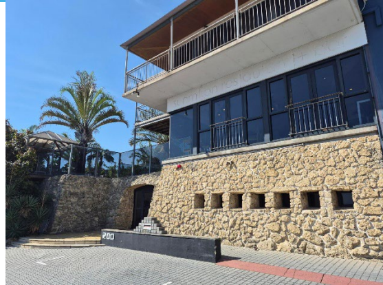
Existing front facade
