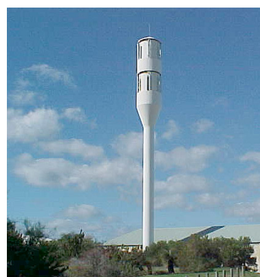
Design and colour of antennas blend with the water tower to which they are attached
