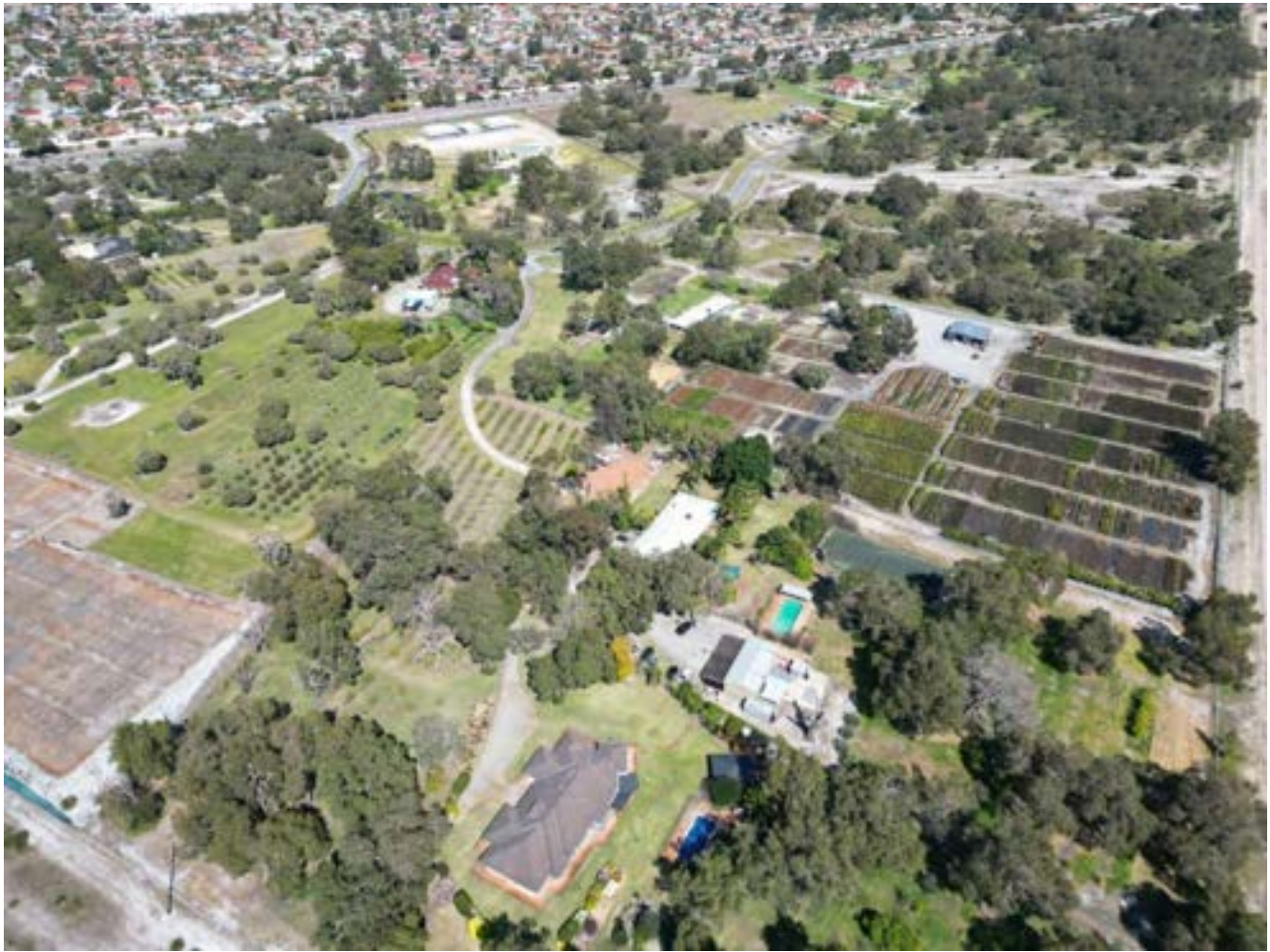
Photograph 4: Aerial view of the site
