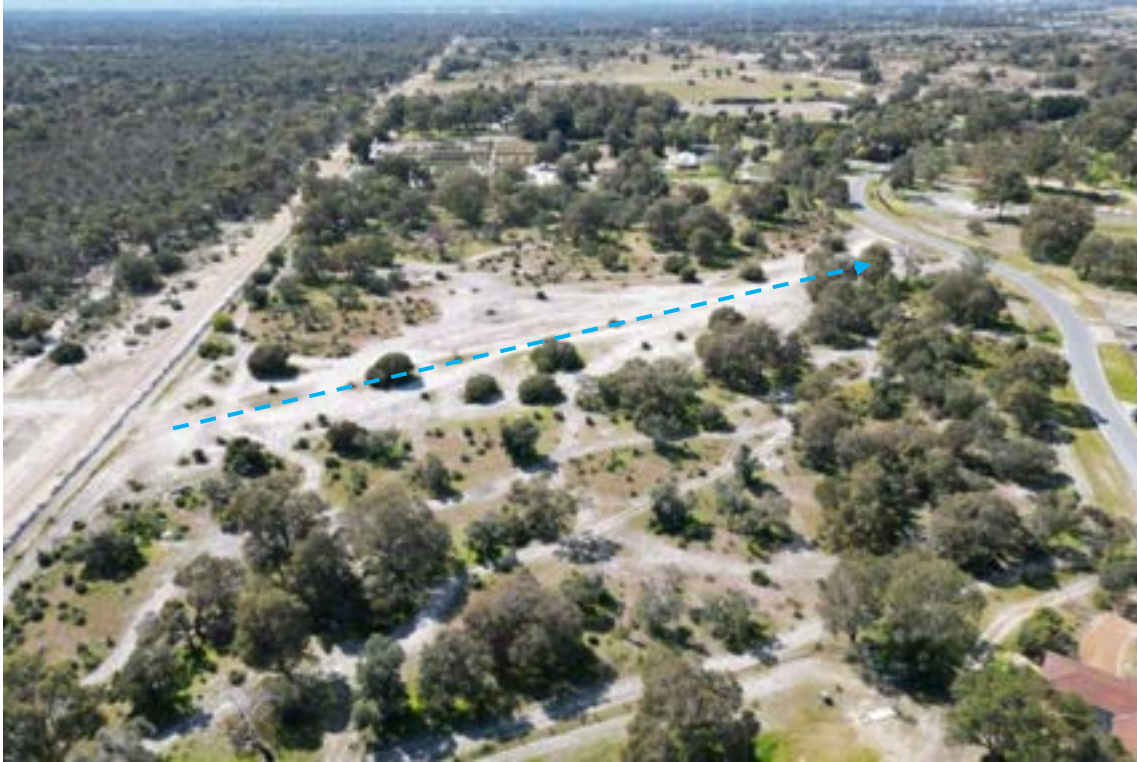
Plate 9: Aerial view. Drain at northern boundary (blue arrow) no longer present. 4WD vehicles activity present. Source of Image: Galt Geotechnics WAG240411-01 001 R Rev0.
