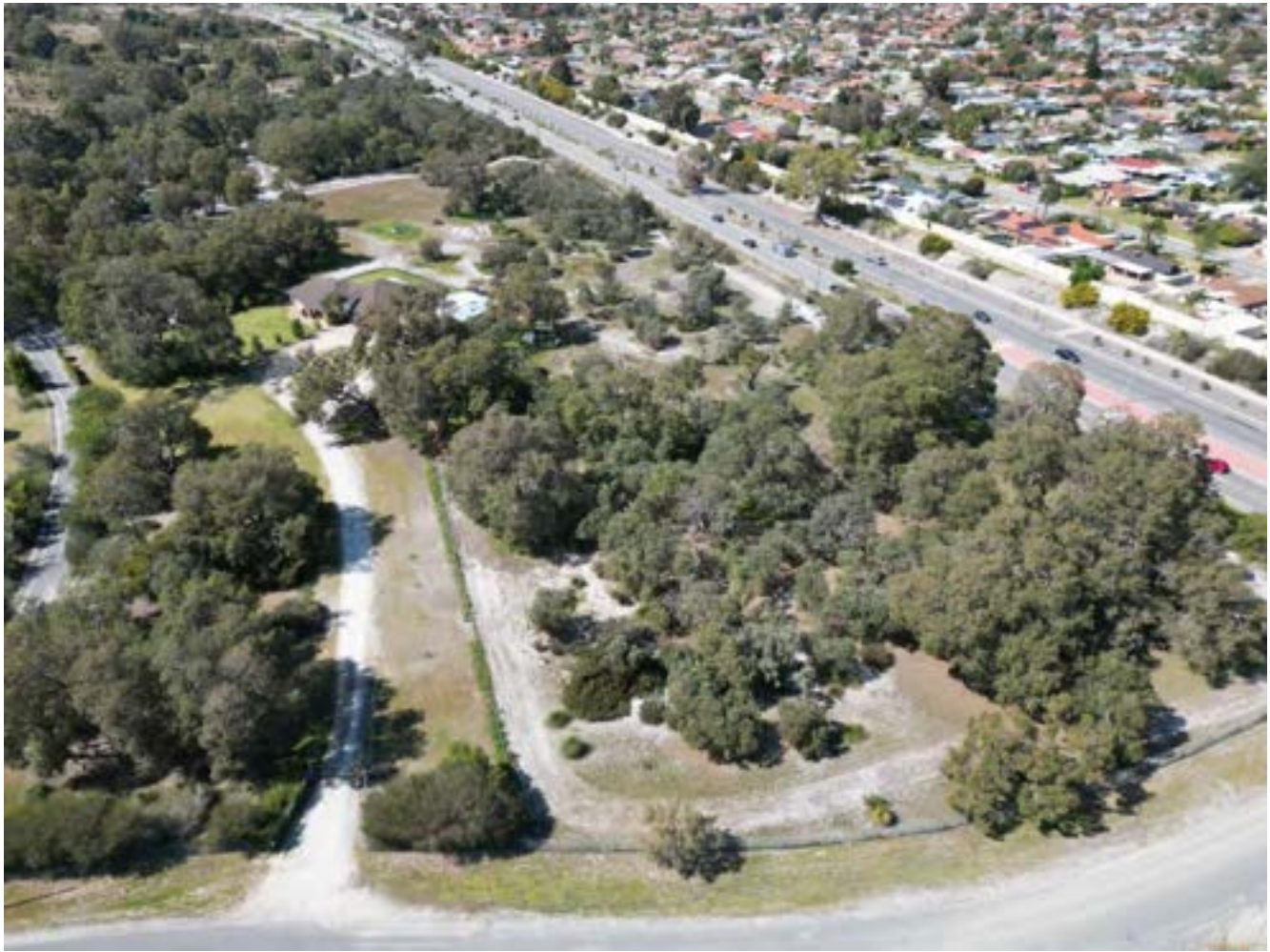
Photograph 3: Aerial view of the site
