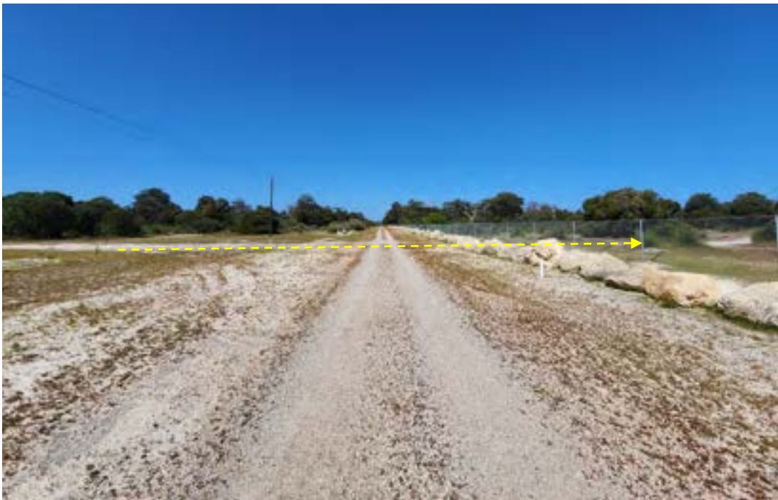
Plate 12: Access track along northern boundary, W-E direction. Yellow arrow shows historical drain pathway, no longer existing. Date of image: 09/10/2024
